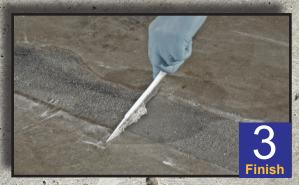
Create a smooth finished surface using a scraper, or trowel. Wait 15 minutes, then turn your floor back to traffic!
