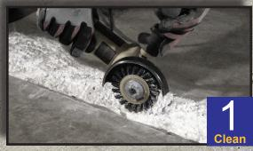
Ensure the repair area is clean and dry. No square cutting or minimum depth requirements.
