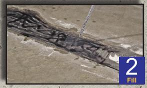
Fill the repair area with clean, washed, and dried sand. Saturate with Rapid Restore.
